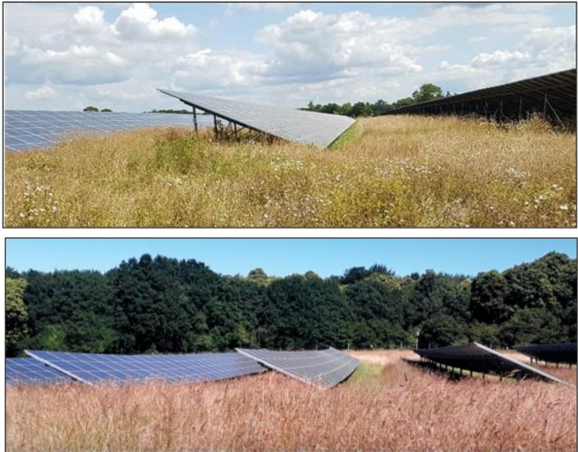
Figure 4.3: Sites where a “Shade Cut” has been employed during the growing season to prevent shading of panels, but allow flowering meadow elsewhere
